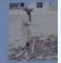
Step 1: Test the soil's permeability. Measure how much water is absorbed in a set time.
